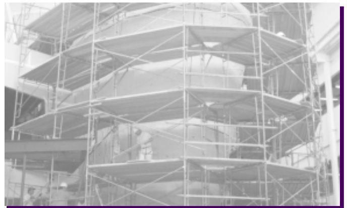
C6 is on schedule for completion in June.
